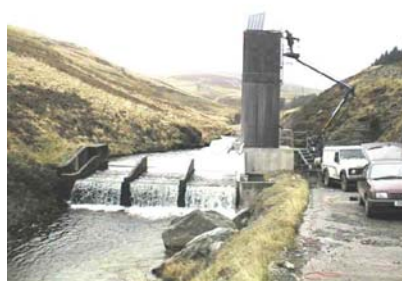
FIGURE 4: Camddwr lime doser, Wales.
