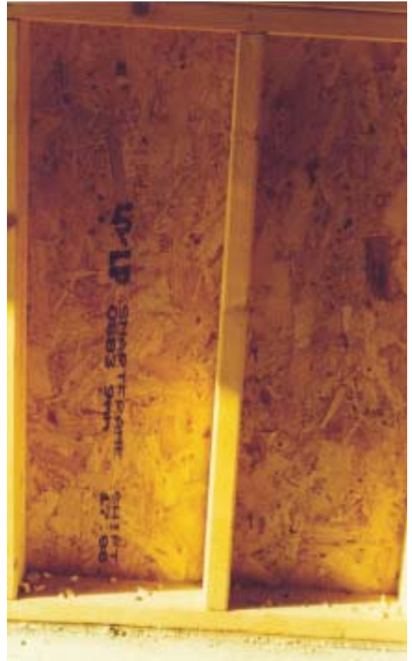
Figure 6: OSB, shown here in a timber frame housing application, is manufactured by Smart Ply Ltd (previously LP Coillte Ltd) in Waterford.
