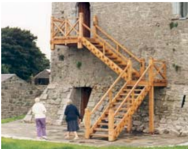
Figure 7: External stairs made from Irish oak at Athenry Castle, Co Galway.
