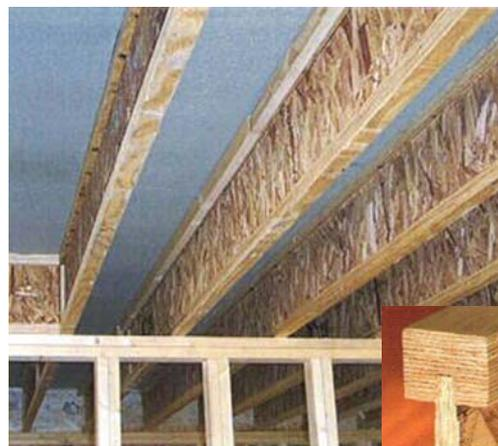
I-beams are being used to replace solid timber in applications such as ceiling joists.
