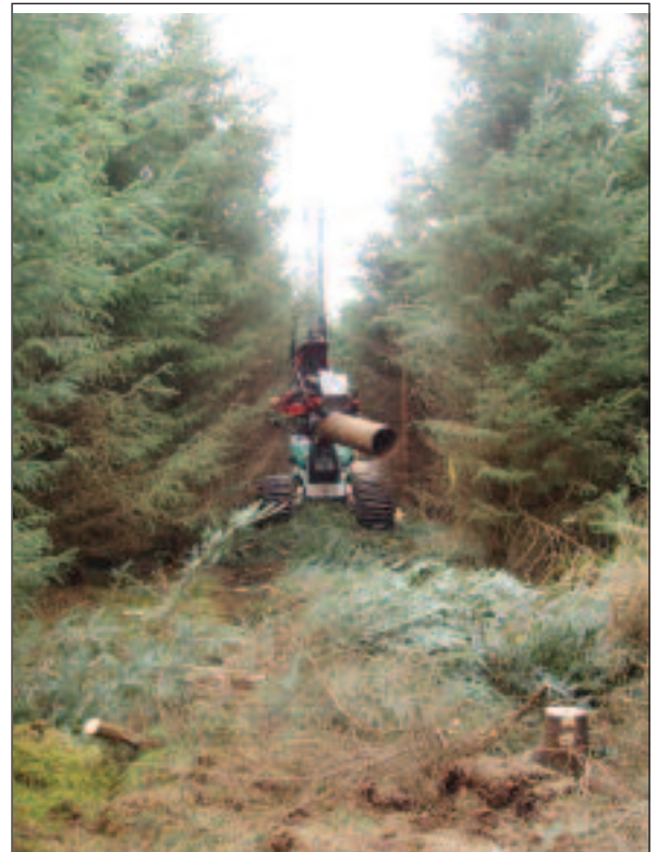
Figure 3: Harvester carrying steel pipe from roadside to drain crossing.
