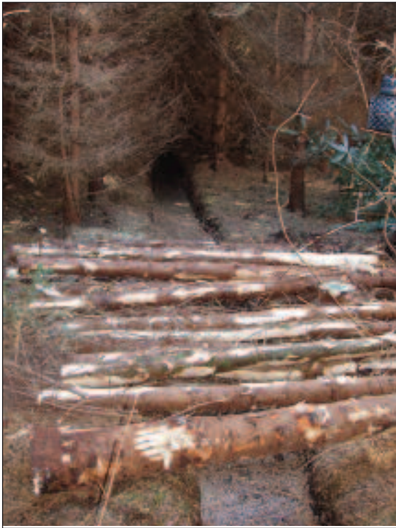
Figure 5: Log bridge under construction.
