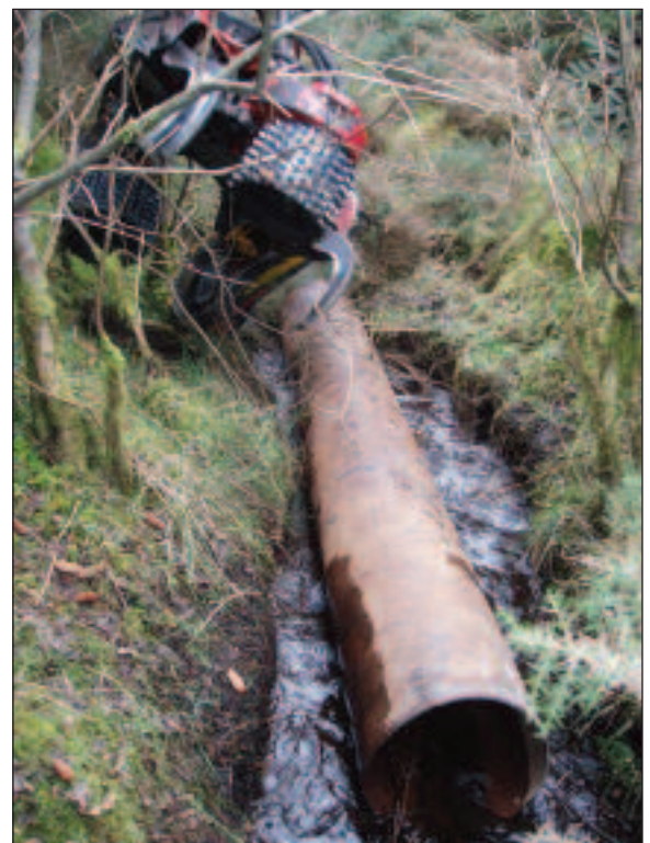
Figure 4: Steel pipe in place in drain.
