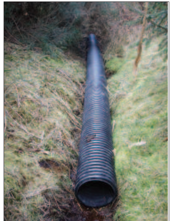
Figure 8: Corrugated plastic pipe in the drain to be crossed.
