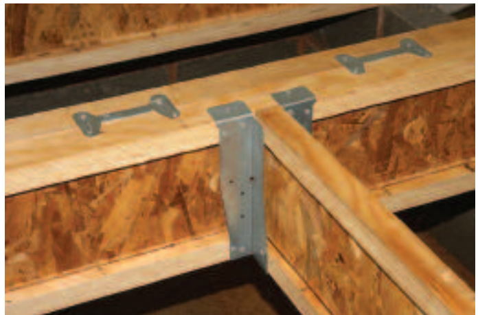
▲ I-beams installed at an Irish construction site.
