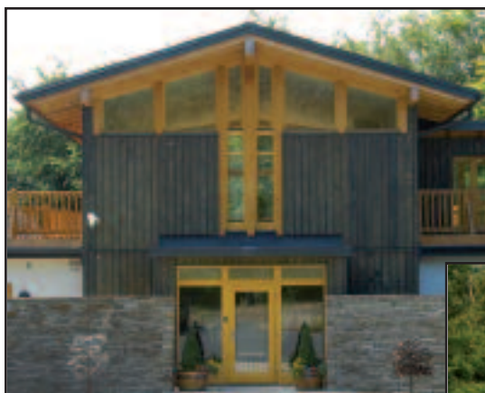
Figure 1: Board on board cladding at Coillte Headquarters.
