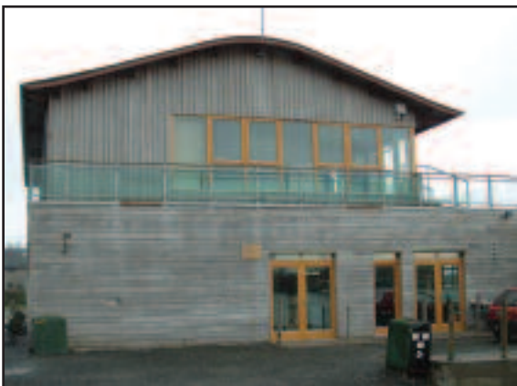
Figure 8: Untreated iroko weathered to a uniform grey – Lough Derg Yacht Club.
