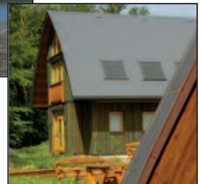
Figure 1: Board on board cladding at Coillte Headquarters.
