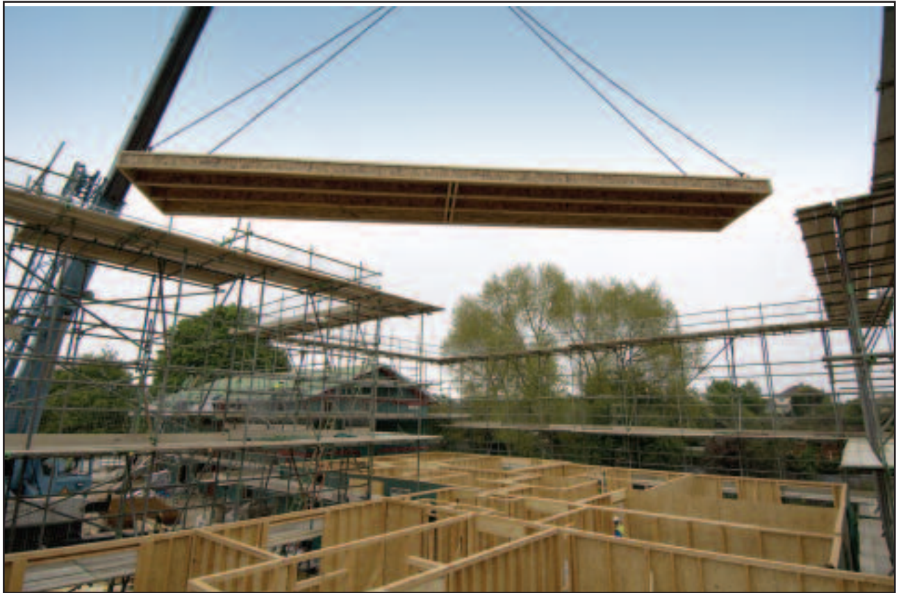
▲ Light-weight floor panels being lifted into position on a timber-frame construction site.
