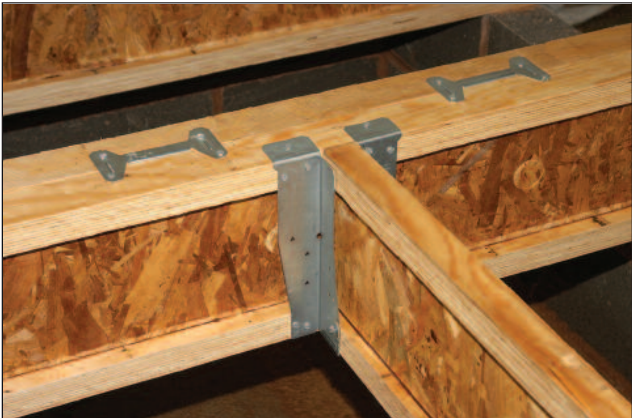
▲ I-joists manufactured from LVL flanges and OSB webs.
