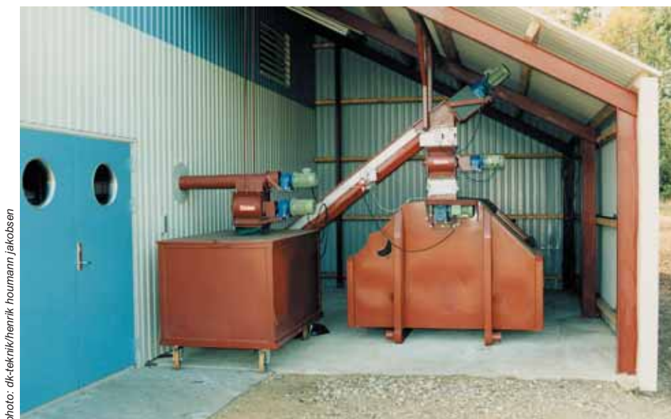
Figure 37: Fly ash from the cyclone is stored in the ash container to the left, while bottom ash from the heating plant is deposited in the large container.
