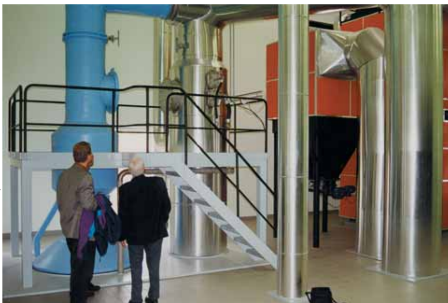
Figure 35: Mist eliminator in brilliant blue and insulating jackets with glittering surfaces situated on the flue gas condenser. The boiler room at Græsted Varmeværk being demonstrated to a foreign visitor look like a "sittingroom".
