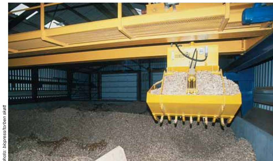
Figure 23: Wood chip storage with crane for the feeding of the wood chip boiler furnace at Harboøre. The crane can be automatically controlled and monitored from a screened control room.
